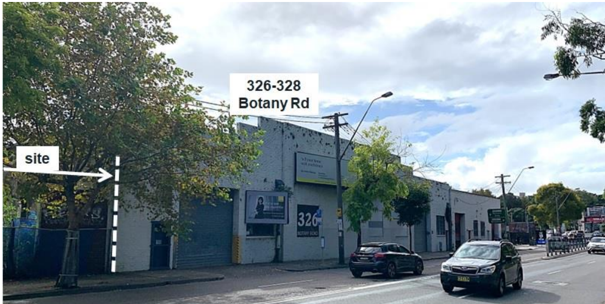
Figure 9: Property at 326-328 Botany Road adjacent to the north of the subject site.
