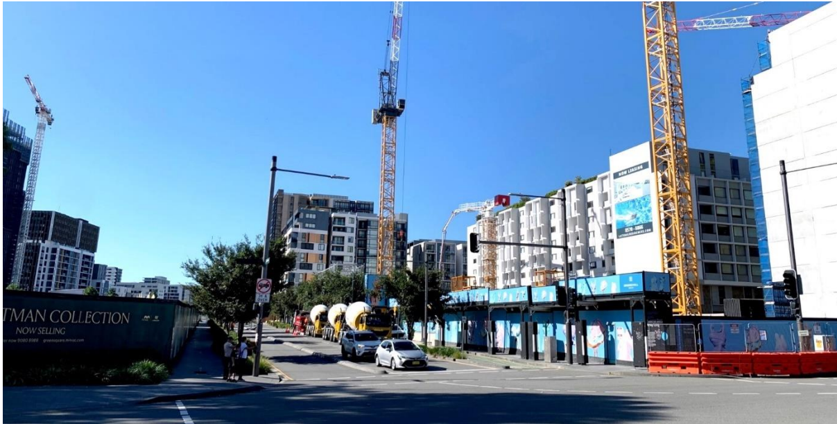
Figure 11: View to Bridgehill mixed use development site at 499 Botany Road.
