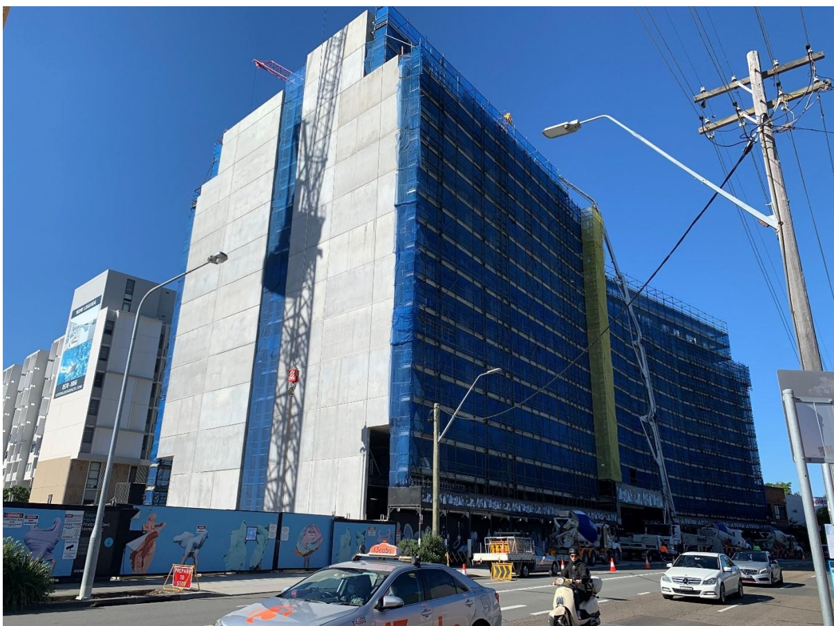
Figure 12: View to Lateral mixed use development site at nos. 501-515 further south on Botany Rd.
