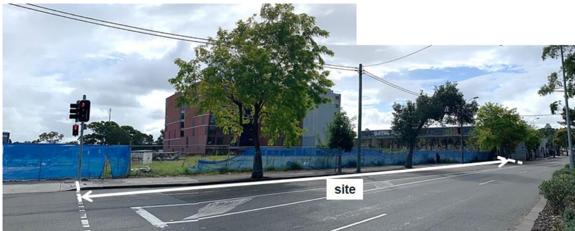
Figure 6: Botany Road frontage of subject site.
