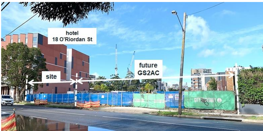
Figure 14: The future GS2AC Road and subject site frontage to O'Riordan Street.
